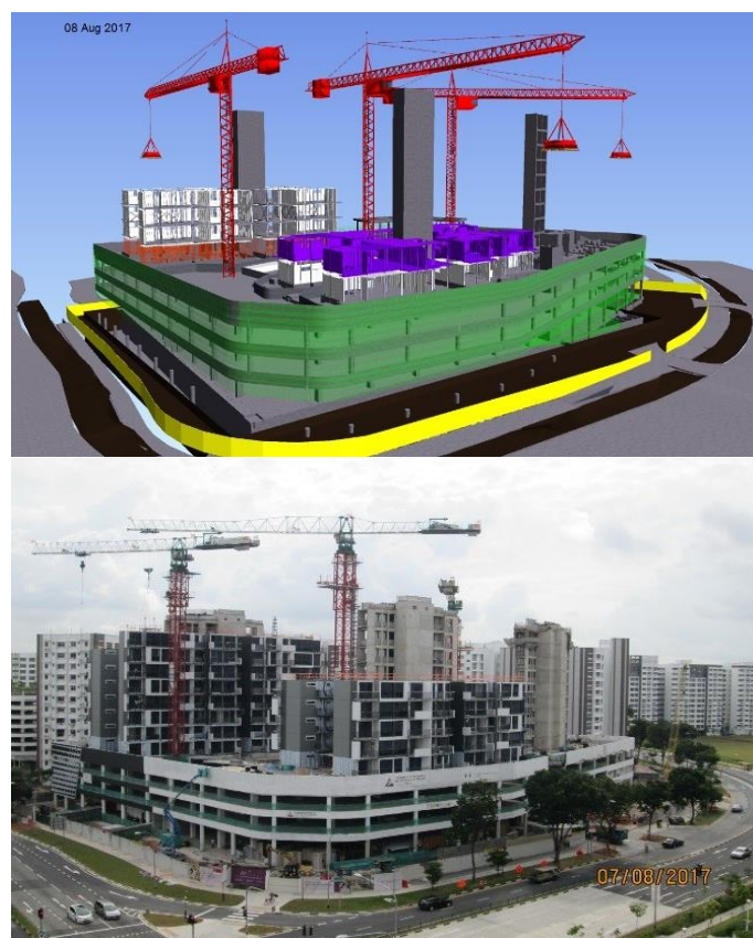
Diagram 2: Planned 4D-BIM vs Actual Progress (Project: Wisteria Mall, Mixed Use Development at Yishun Avenue 4, Singapore)
