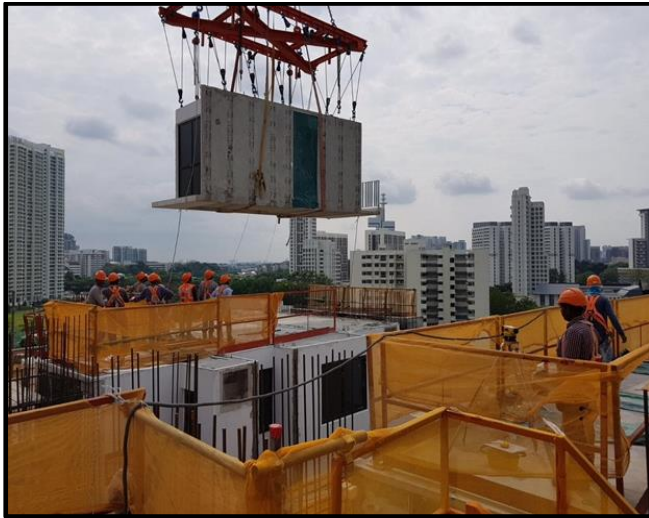
PHOTO 1: PPVC INSTALLATION IN PROGRESS
