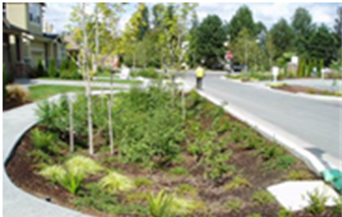
Roadside Bioretention Swale (LID) (Source: City of Kirkland)
