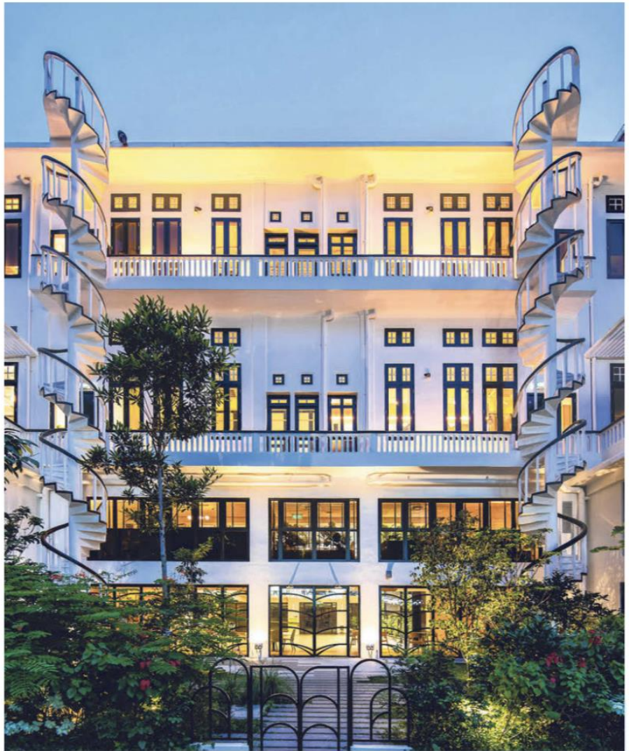
The conservation of Temasek Shophouse in Orchard Road started in 2018 and took 18 months to complete. PHOTO: SURBANA JURONG
